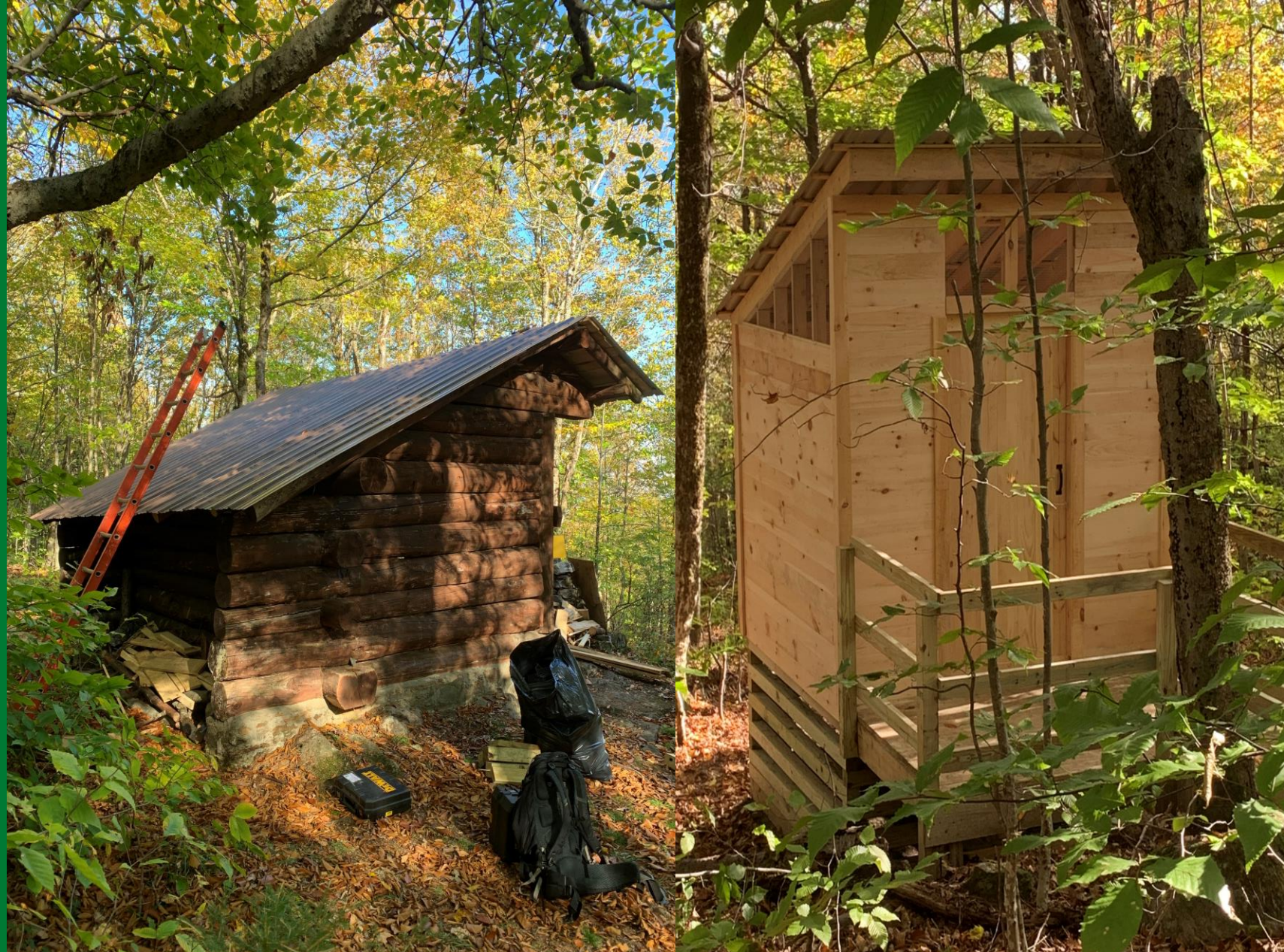
Coolidge State Forest, West - Russell Hill shelter roof repair and privy replacement
